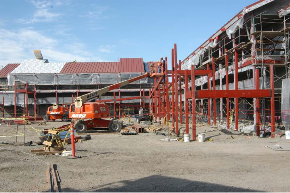
Building C and D – Two Story Classrooms
