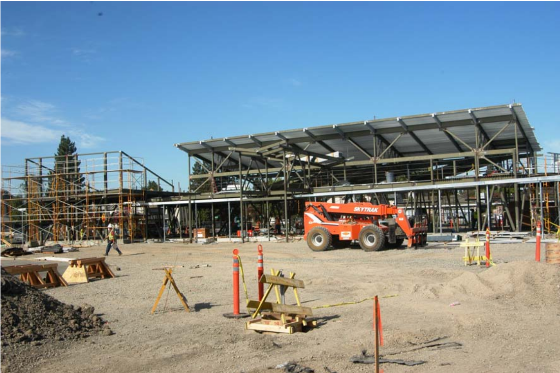
Library Steel Frame and Deck
