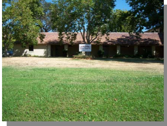
West Wing Roof at A. Warren McClaskey
