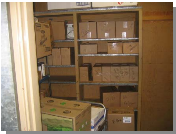
Wood Shelving in Dry Food Storage - Health Code Violation at Freeport Elementary and Multiple School Sites
