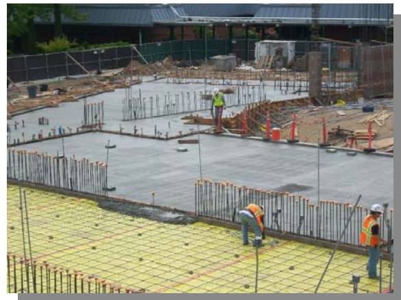
Slab Placement in Progress
