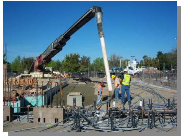
Crushed Rock Installation
