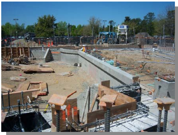
Concrete Wall at Stage
