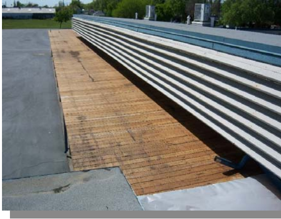
Roofing at Mark Twain ES
